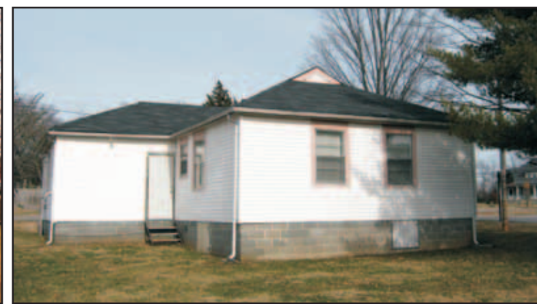
VIEW OF REAR - 416 HILLCREST STREET
